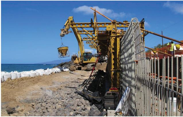
Fig. 3.2f—Construction of seawall with GFRP bars.
